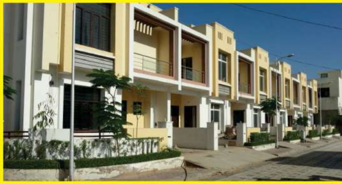
Mehak निर्माण Rudrapur, (Delivered in year 2011)
