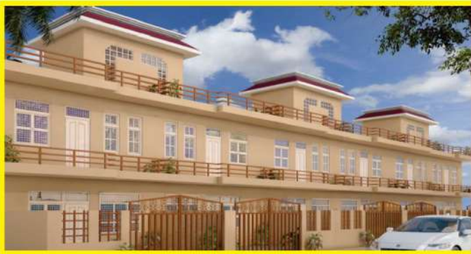
Mehak Eco City (100 Sq. Yd. Villas) NH-91, G.T. Road, Ghaziabad (Delivered in year 2017)
